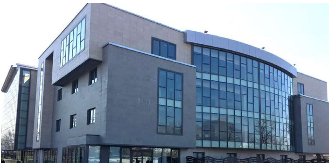
» Overall view of completed structure.
