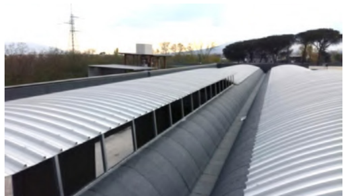
» Roofing between 'PRISMA' elements with Sandwich Panel - External view
