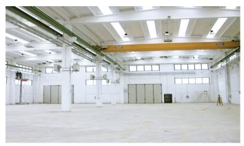
A system that identifies a decades-long tradition of prefabrication in northern Italy, the double-slope beam remains to this day the optimal solution for numerous building types.
