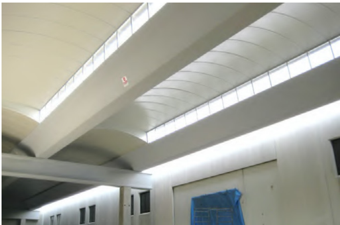
» Roofing between 'PRISMA' Elements with Sandwich Panel - Inside View
