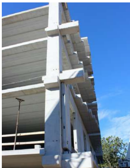
» STRATOS Multi-Storey Structure with Overhangs and Panels
