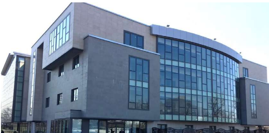
» Overall view of completed structure.
