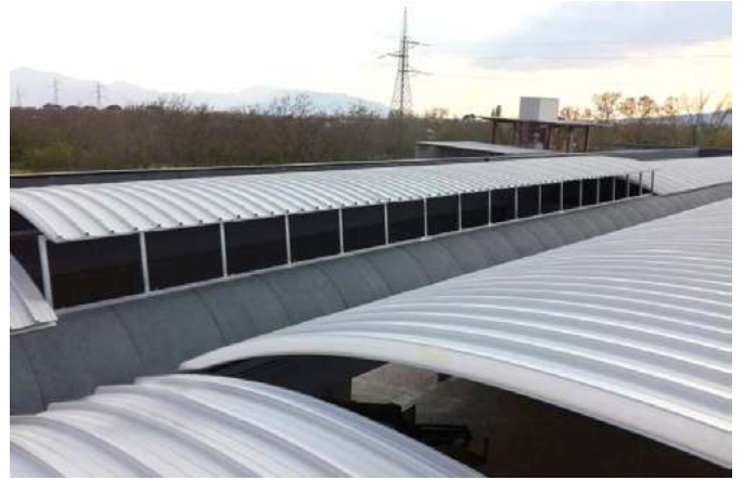
» Roofing between 'PRISMA' Elements with Sandwich Panel - External View
